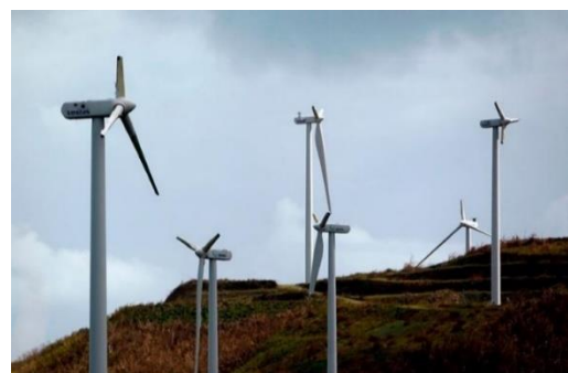
Figure 3 The state of wind turbines after a hurricane. This is what happens when the wind reaches Category 3 hurricane-level wind speeds of 178-208 km/h. There is also Category 4 and 5 which reaches up to 257 km/h wind speeds.
