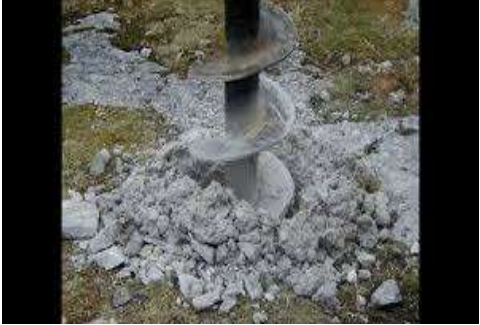
SCREW PILE FOUNDATION
